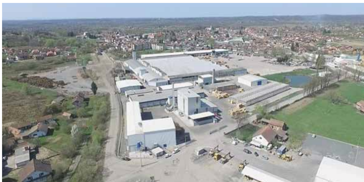
Figure 3.5 – Aerial view of the Glina cogeneration plant Source: adapted from http://sherif.hr/
